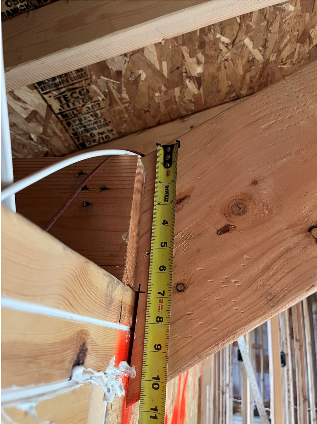
Notched rafters above great room
