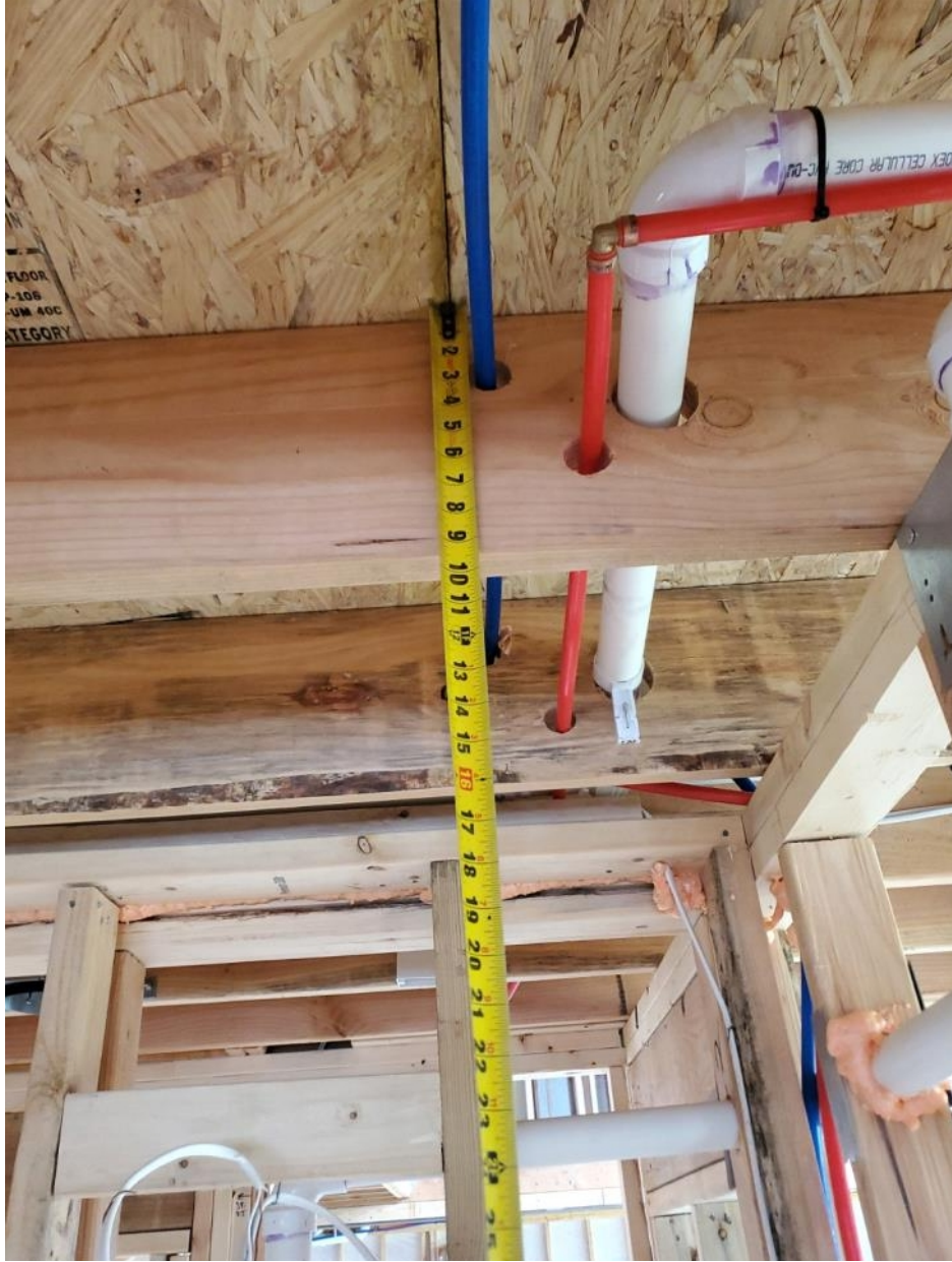
JOIST PENETRATIONS BETWEEN MASTER SUITE/BATH
