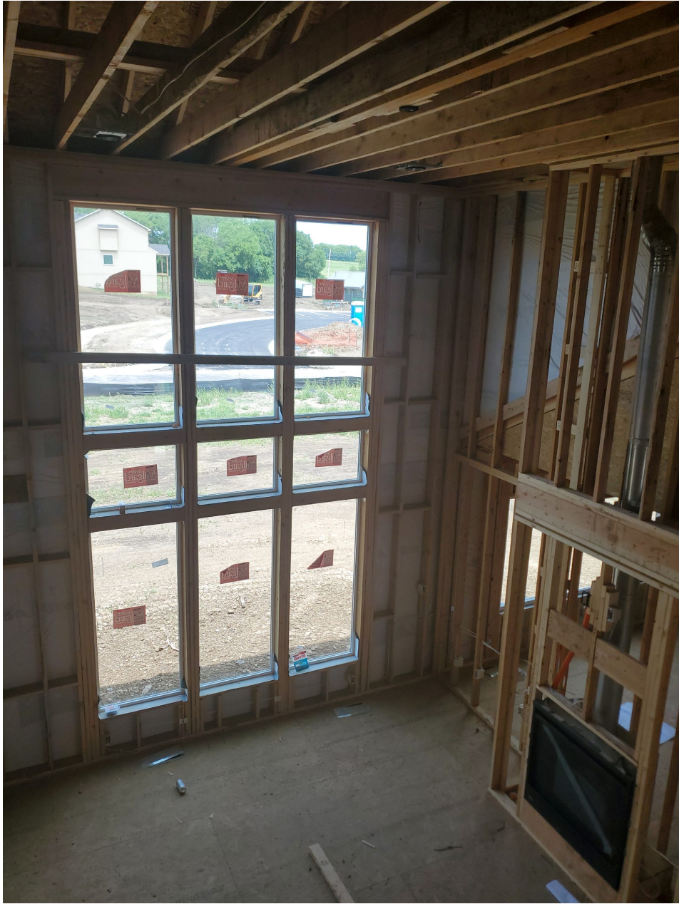
HEADER FRAMING AT GREAT ROOM
