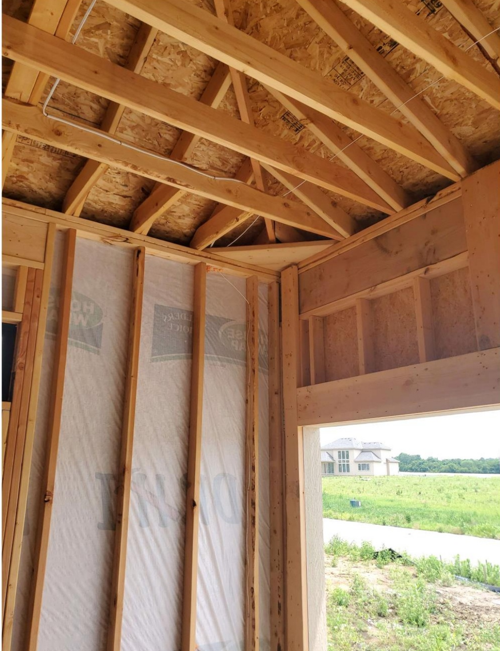
HIP RAFTER AT GARAGE
