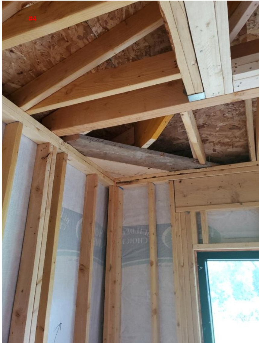
RAFTER/CEILING JOIST AT MASTER SUITE
