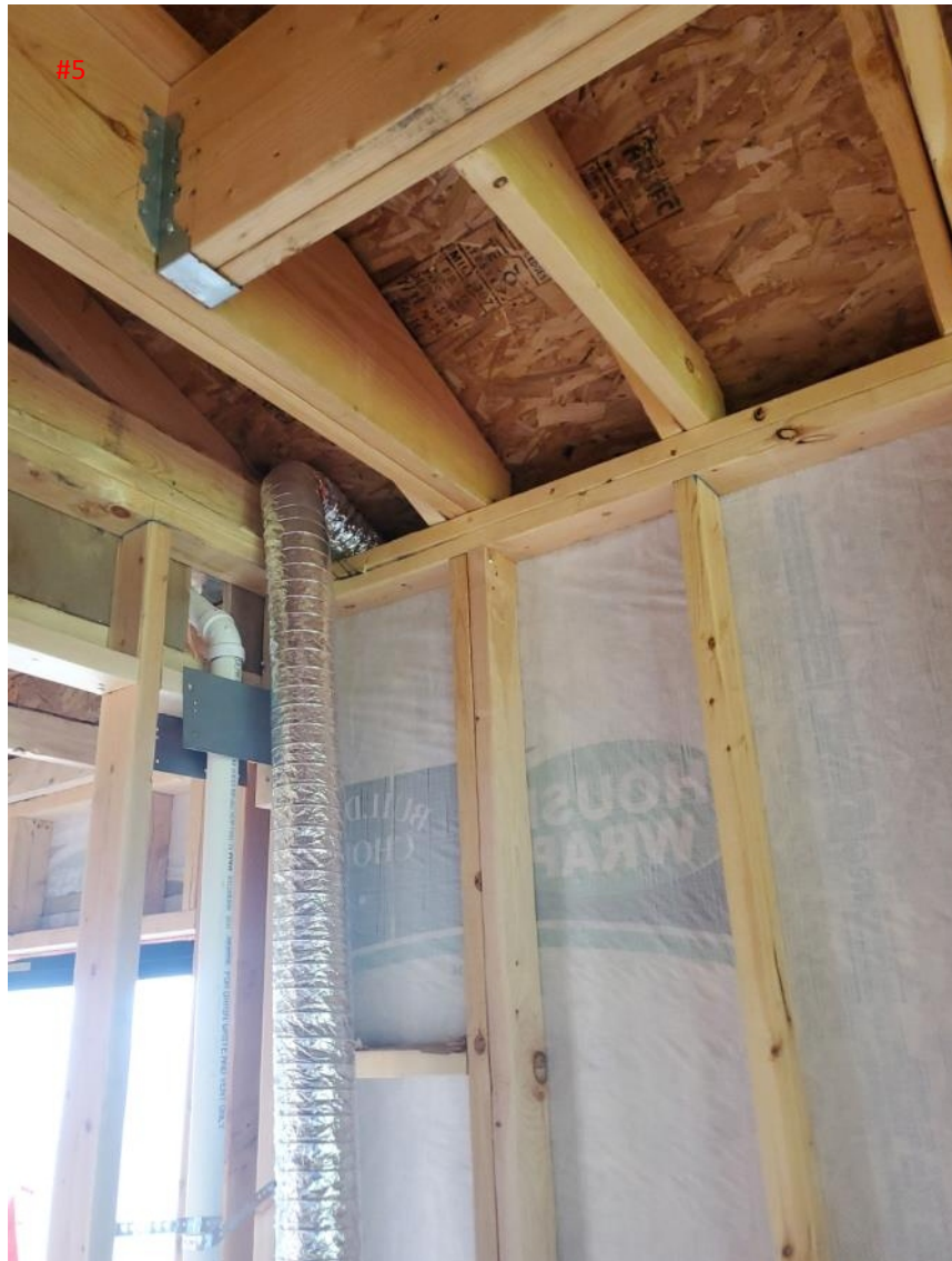
CEILING JOIST/BM AT MASTER BATH
