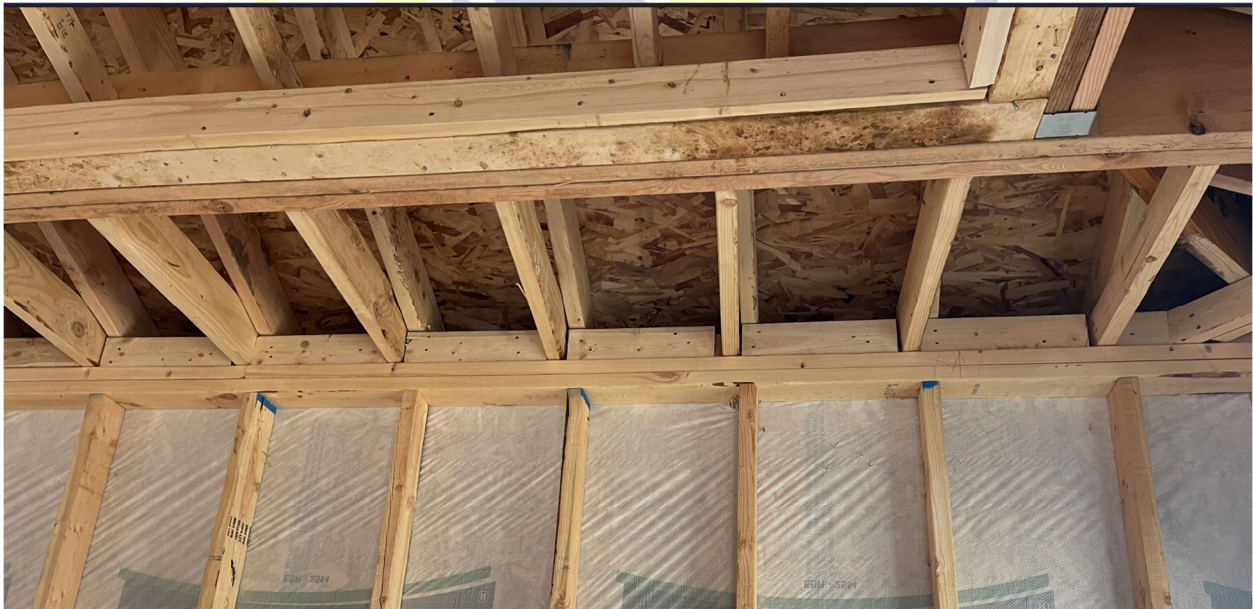
Figure 2 – Rafter framing on blocking between ceiling joists (item 1)
