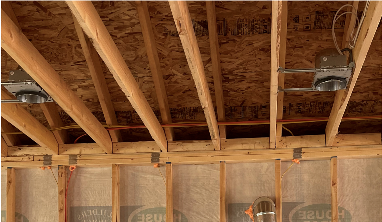
Figure 1 – Rafter framing on blocking between ceiling joists (item 1)
