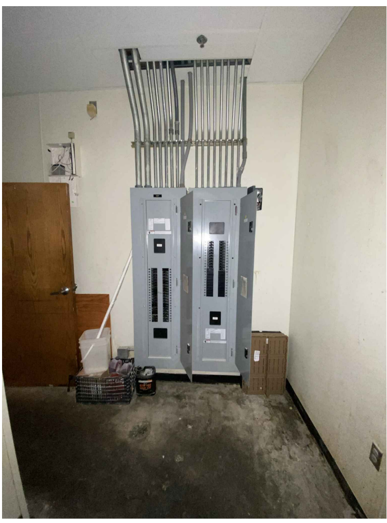
3 EXISTING TENANT PANELS "MDP" PHOTO #2 SCALE: NONE
