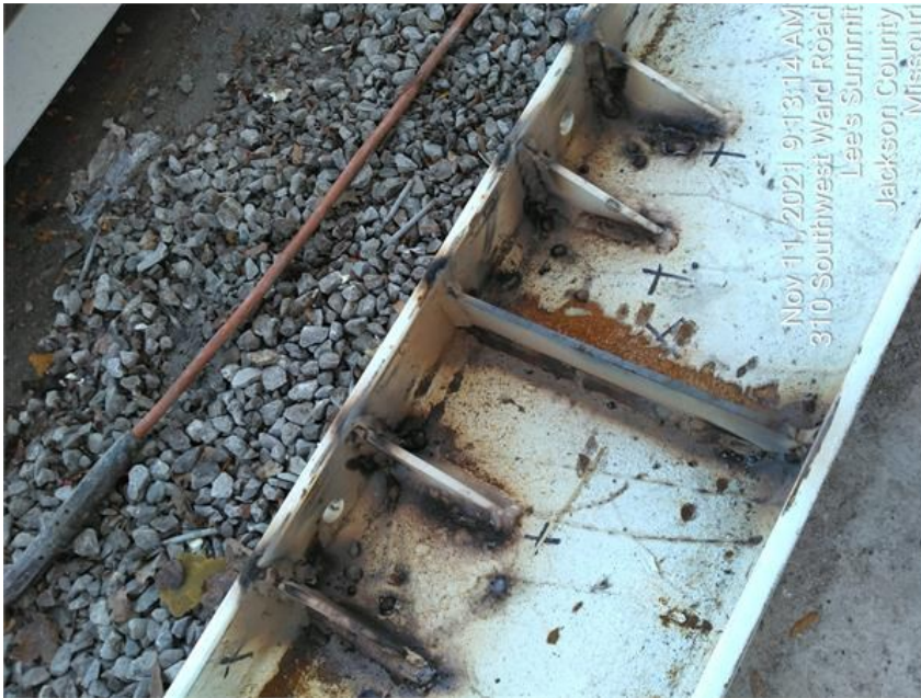
Weld repairs acceptable
