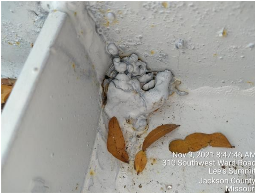
Unacceptable welding – Cold Lap, Incomplete Fusion, & Weld Profile
