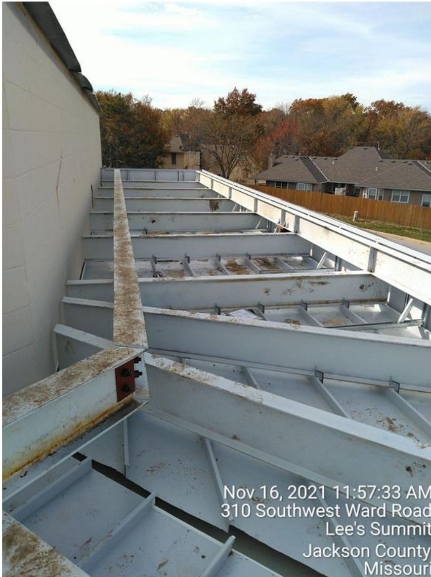
Structural members repaired
