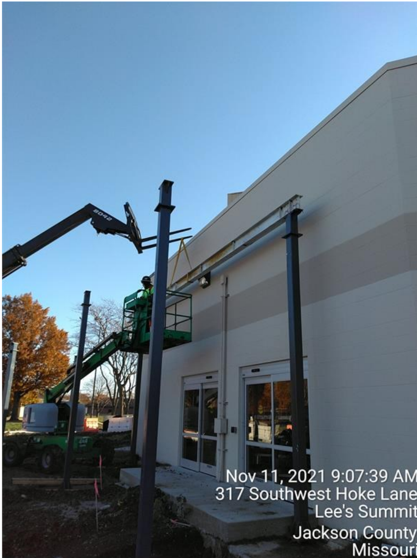
Repaired beam erected on acceptable column
