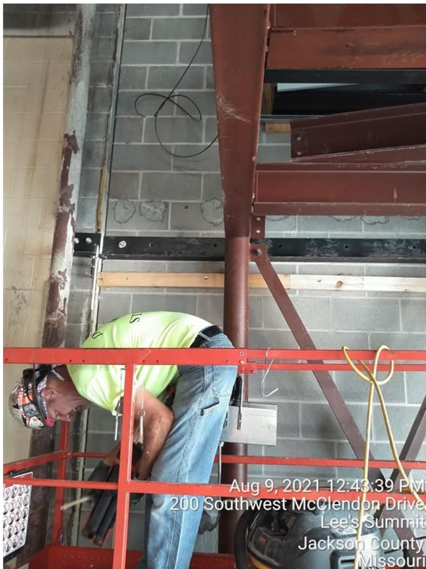
Lateral anchors in lintel angle above door
