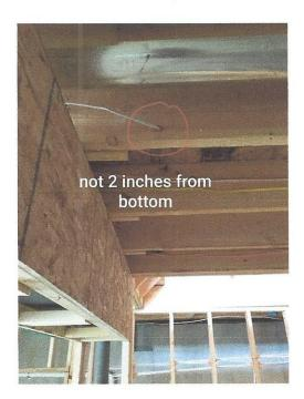
To correct this condition you should install a 1.5" wide x about 18" long metal strap at the bottom of the floor joist approximately centered under the hole that was drilled by the electrician. This will strengthen the bottom of the joist and more than make up for any strength lost by drilling the hole.
