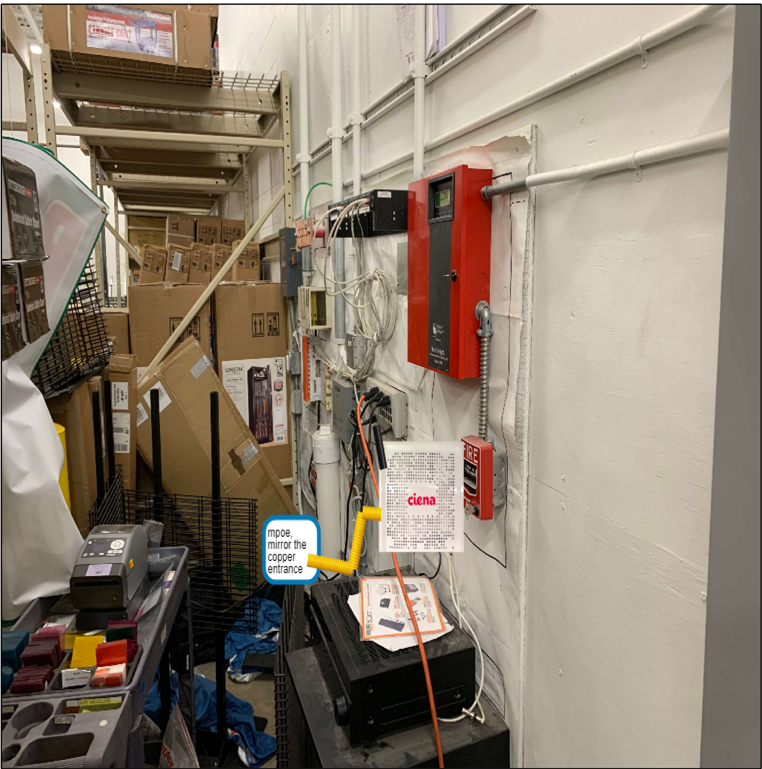
NORTH INTERIOR WALL
