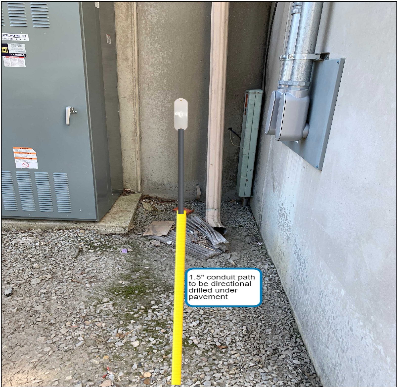
NORTH EXTERIOR WALL
