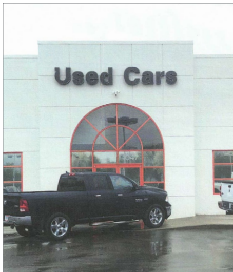
EXISTING SIGN (to be Removed)
