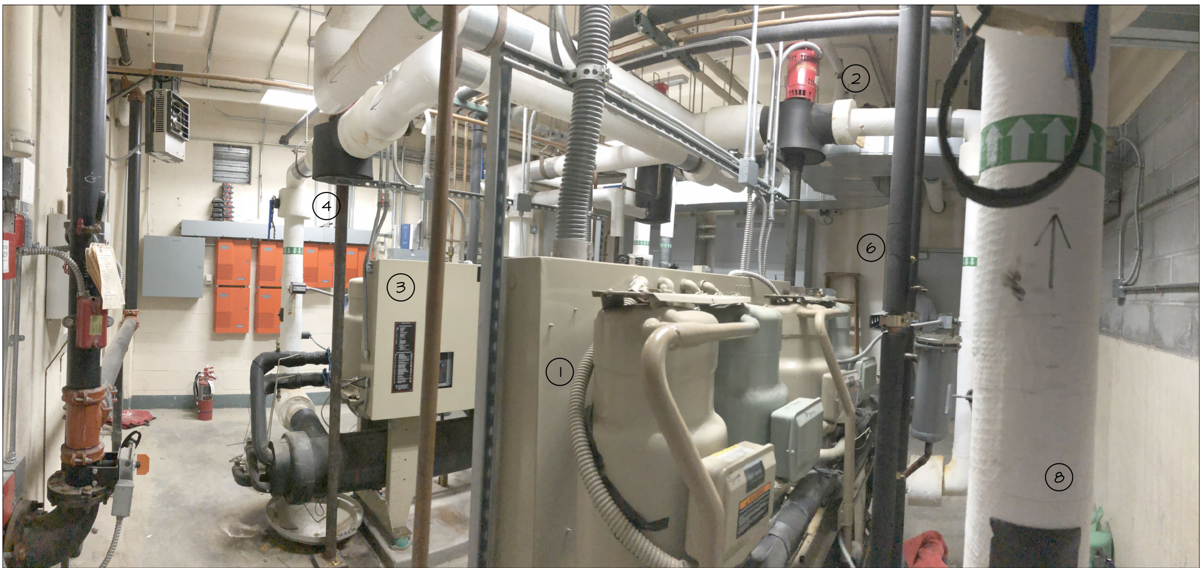
EXIST. CONDITION PHOTO #3
