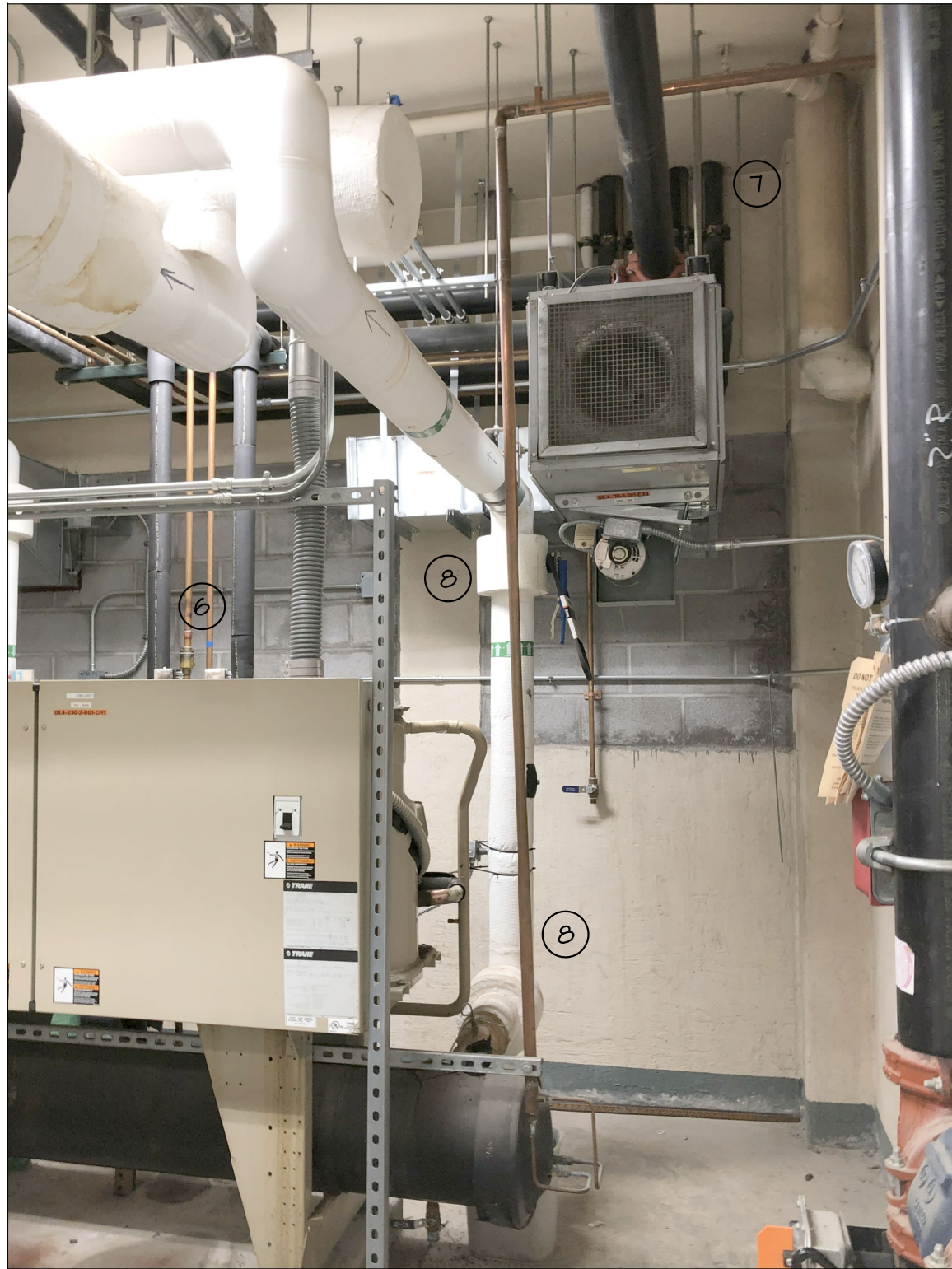
EXIST. CONDITION PHOTO #9
