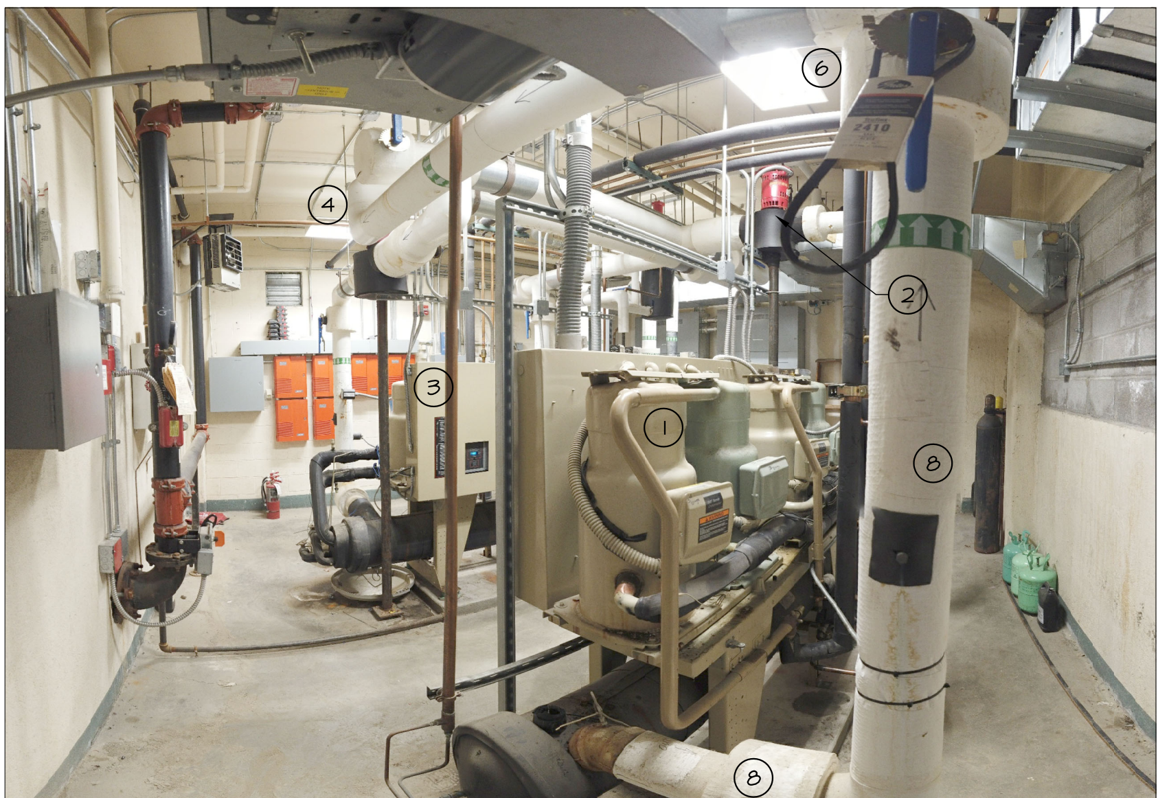
EXIST. CONDITION PHOTO #4
