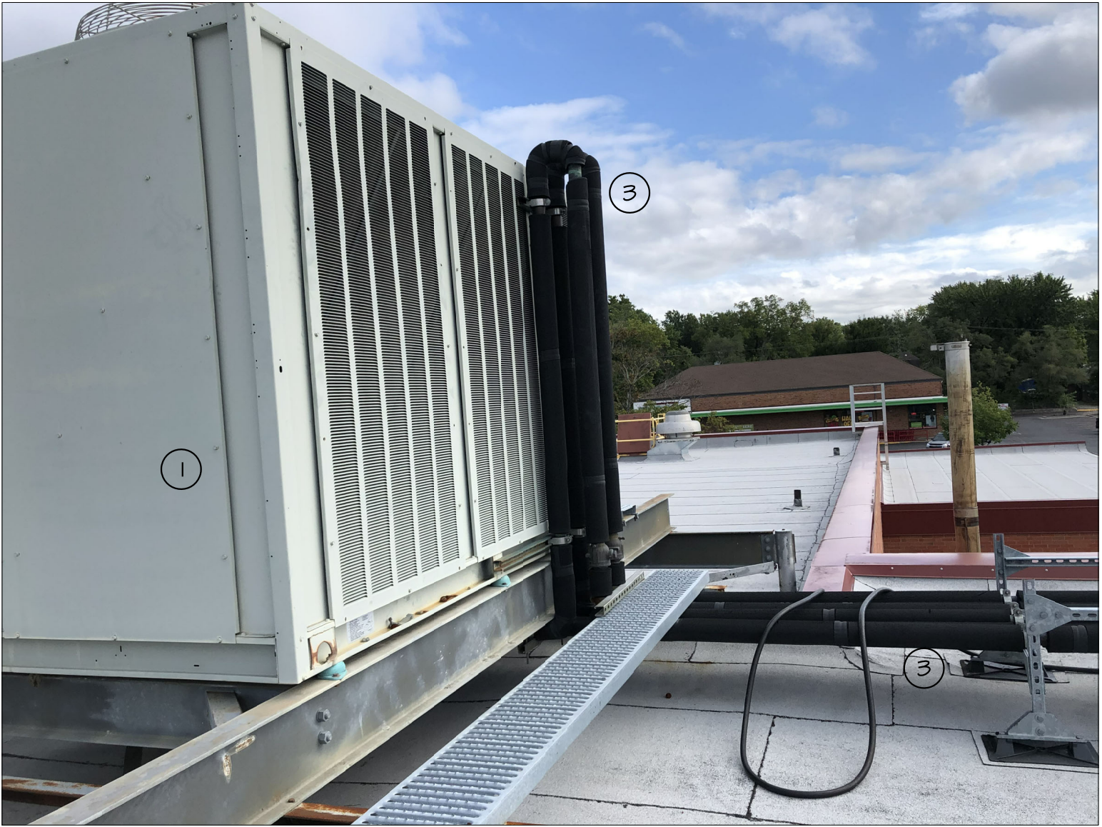
EXIST. CONDITION PHOTO #20
