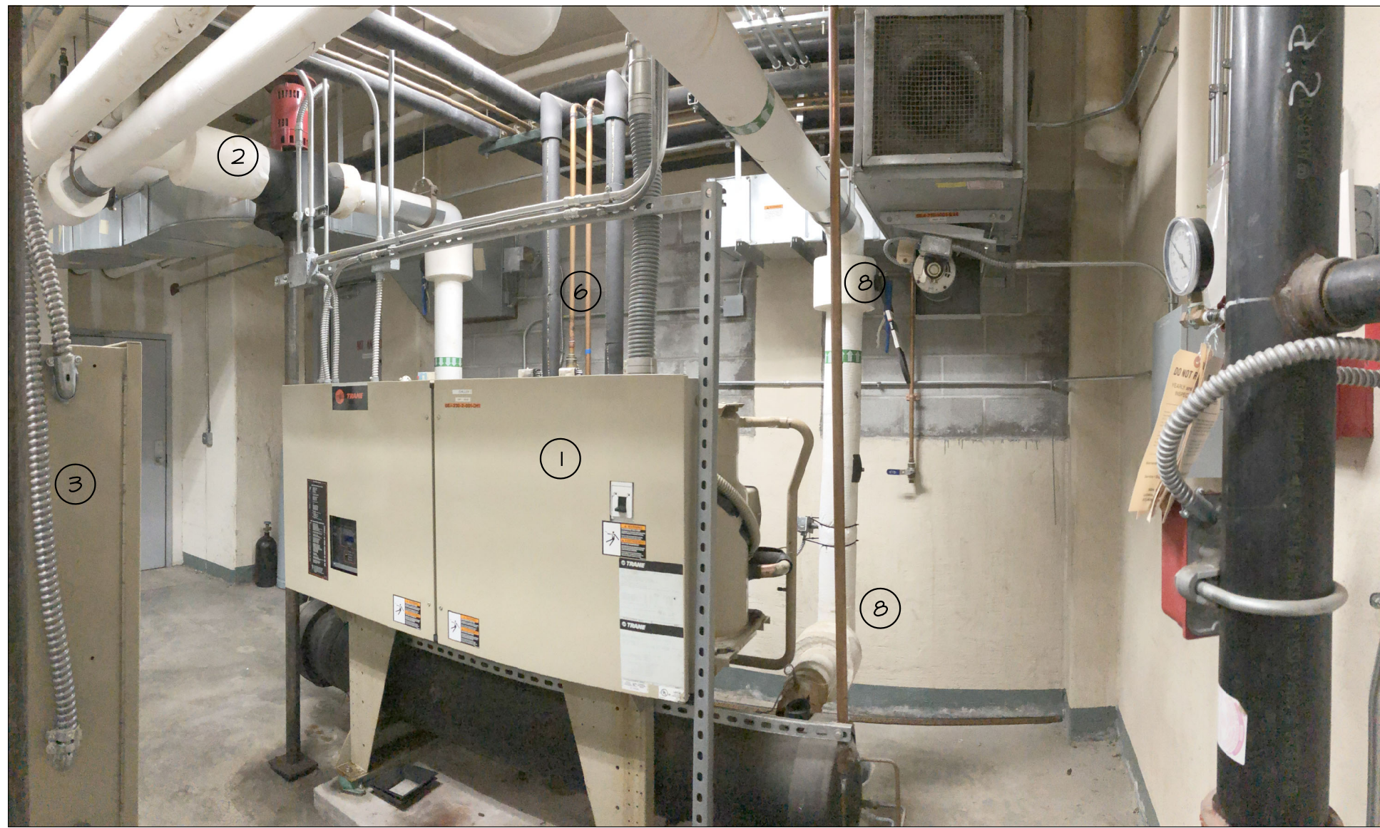
EXIST. CONDITION PHOTO #1
