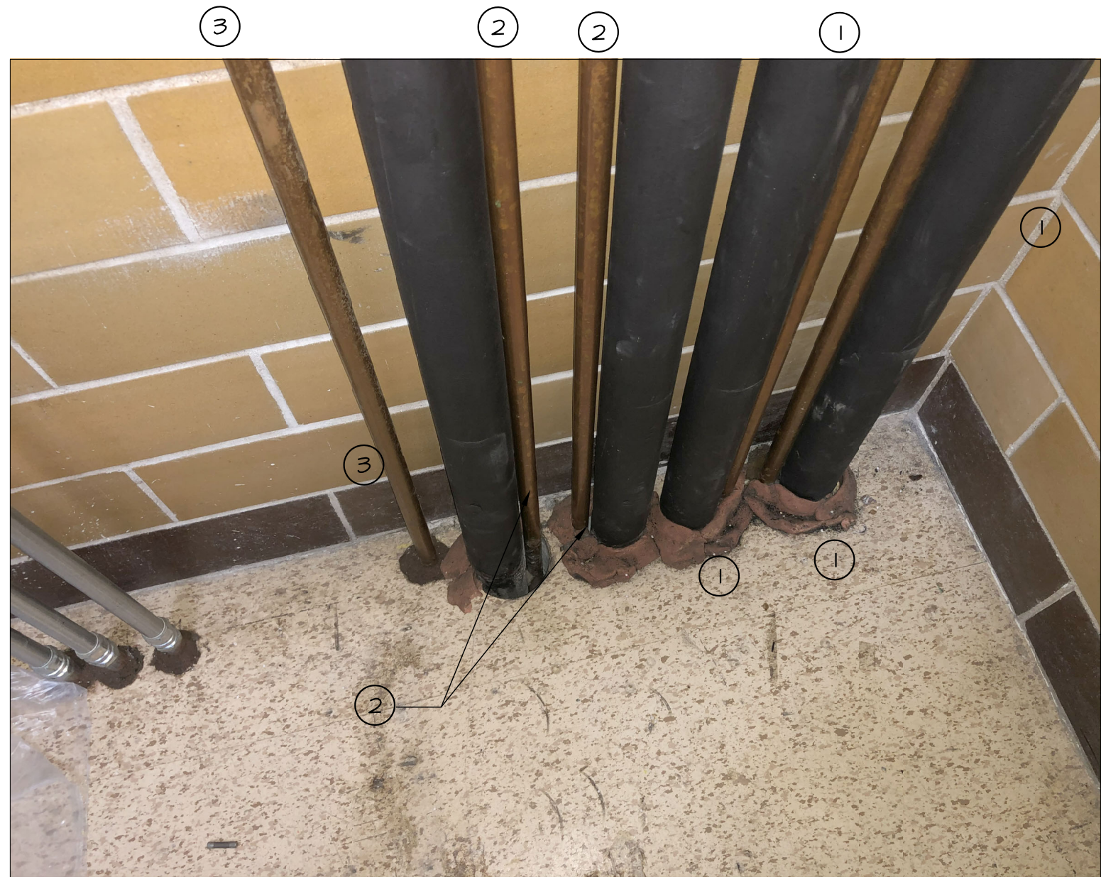
EXIST. CONDITION PHOTO #10
