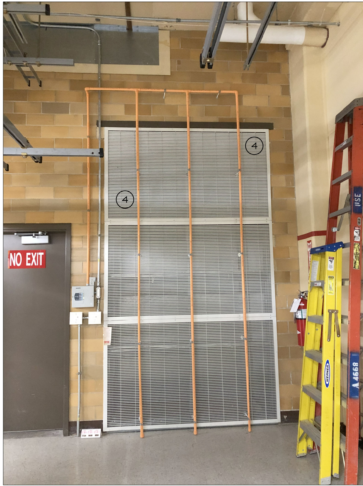
EXIST. CONDITION PHOTO #13
