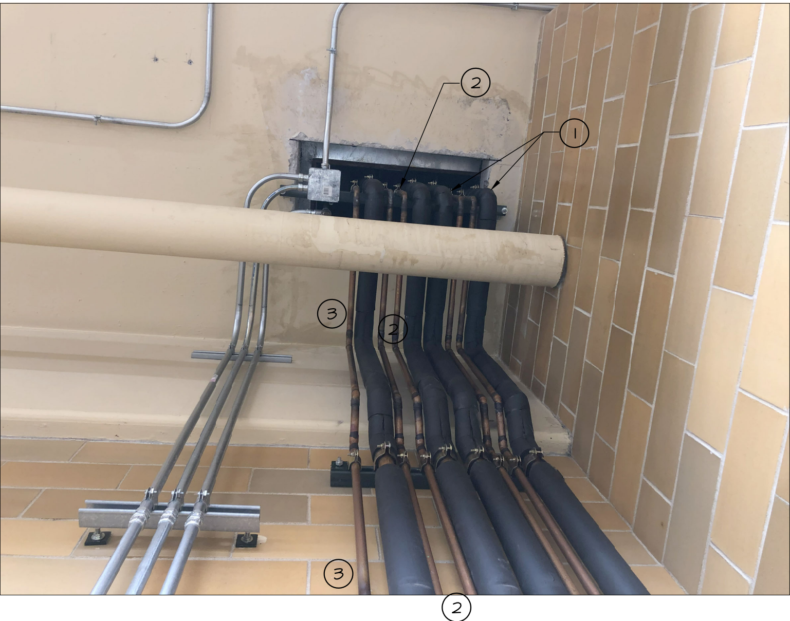
EXIST. CONDITION PHOTO #12
