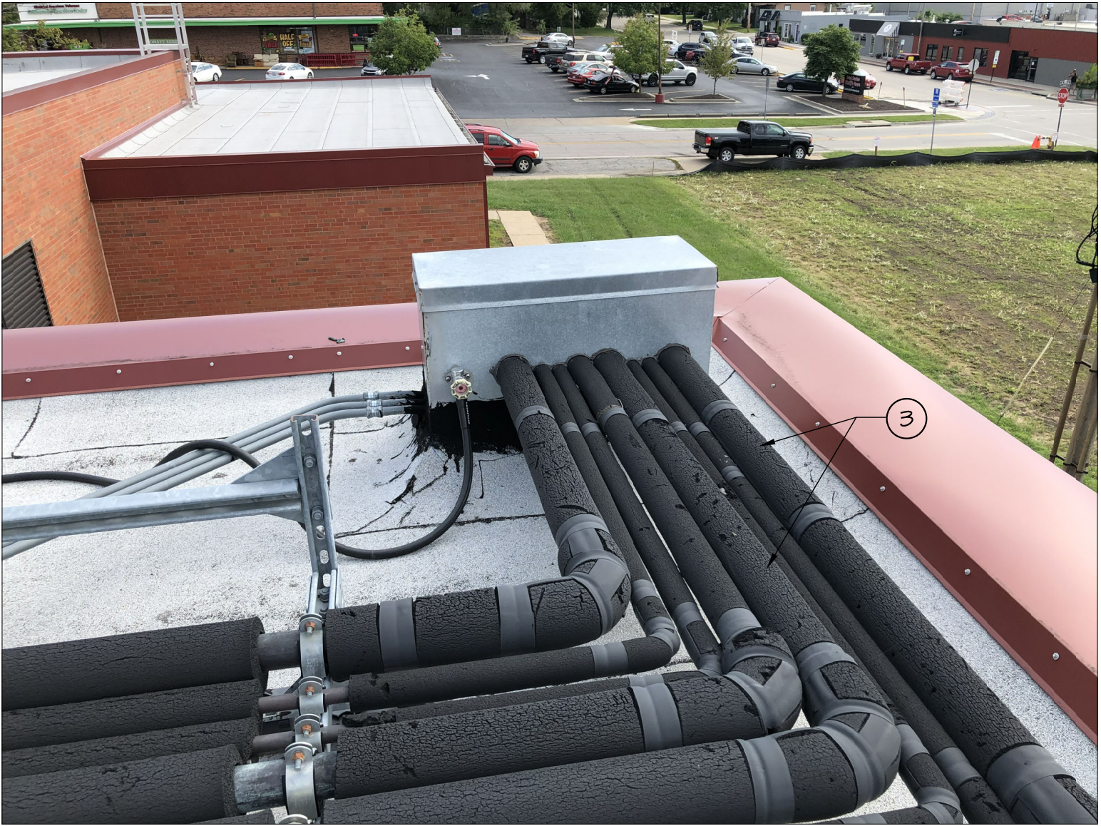
EXIST. CONDITION PHOTO #21
