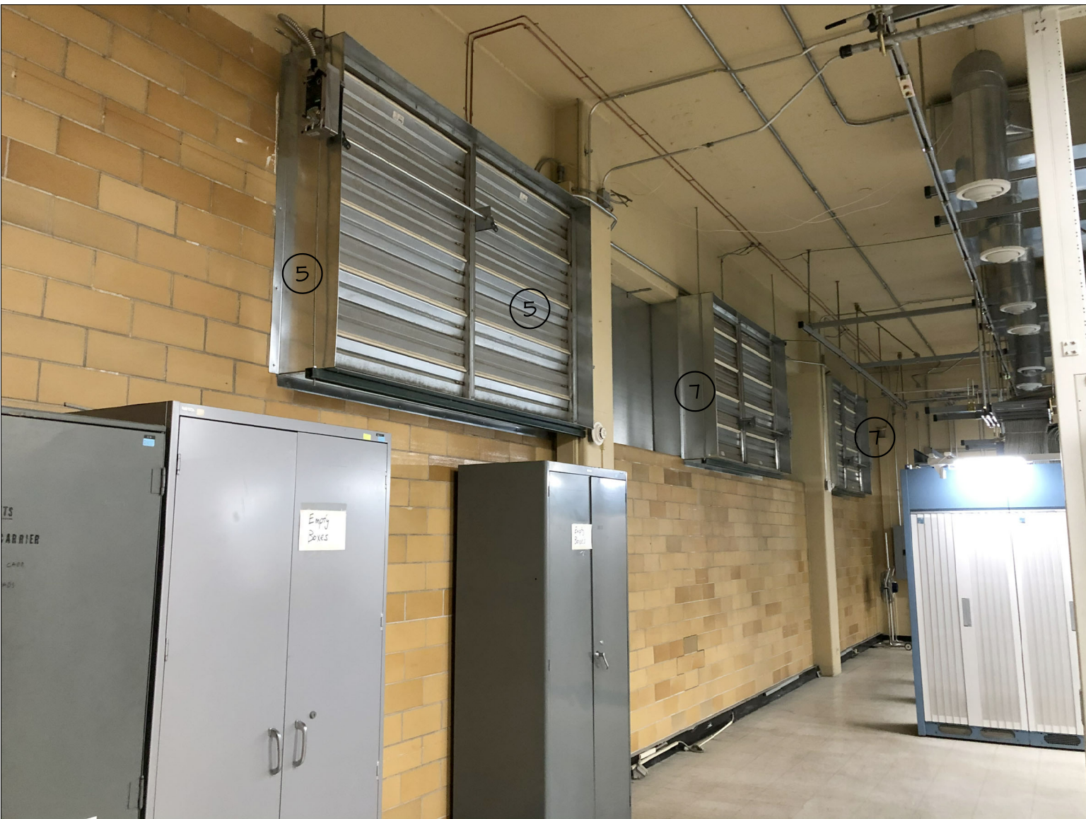
EXIST. CONDITION PHOTO #14
