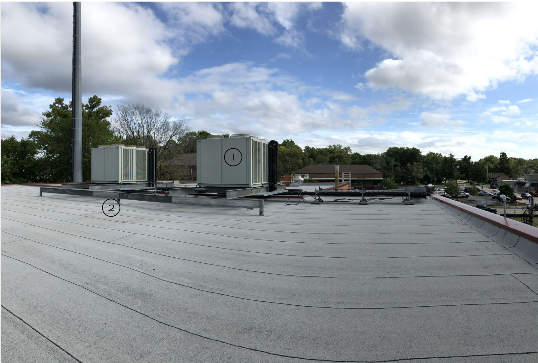
EXIST. CONDITION PHOTO #17
