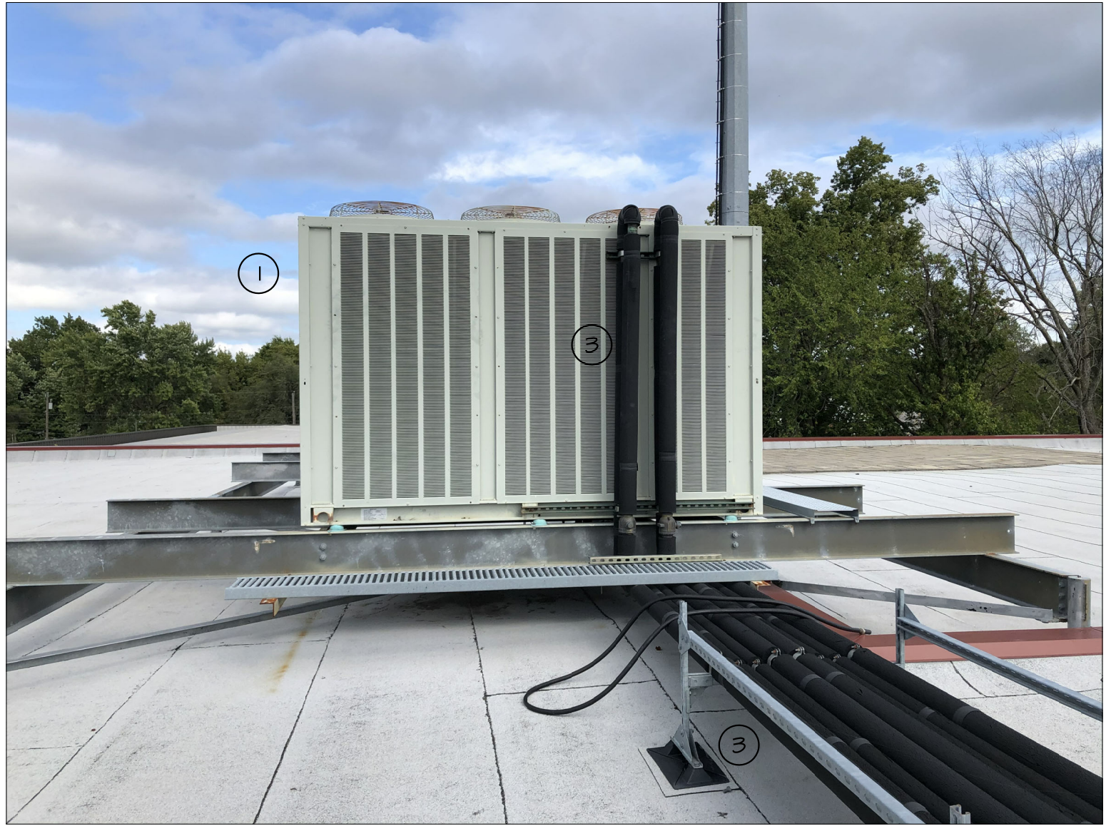
EXIST. CONDITION PHOTO #19
