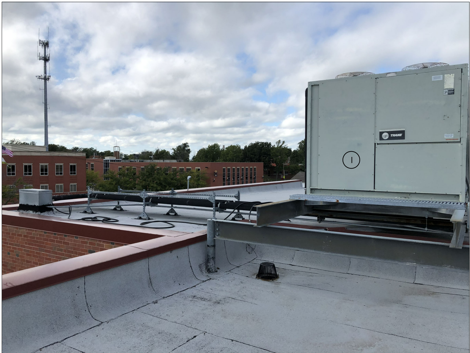
EXIST. CONDITION PHOTO #18
