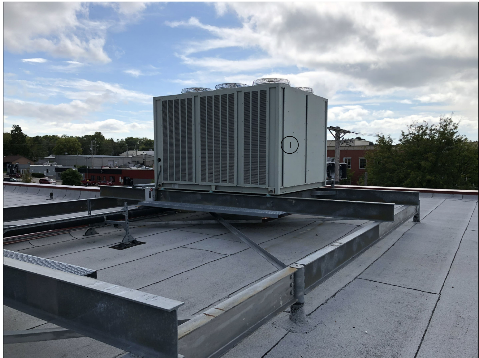
EXIST. CONDITION PHOTO #16
