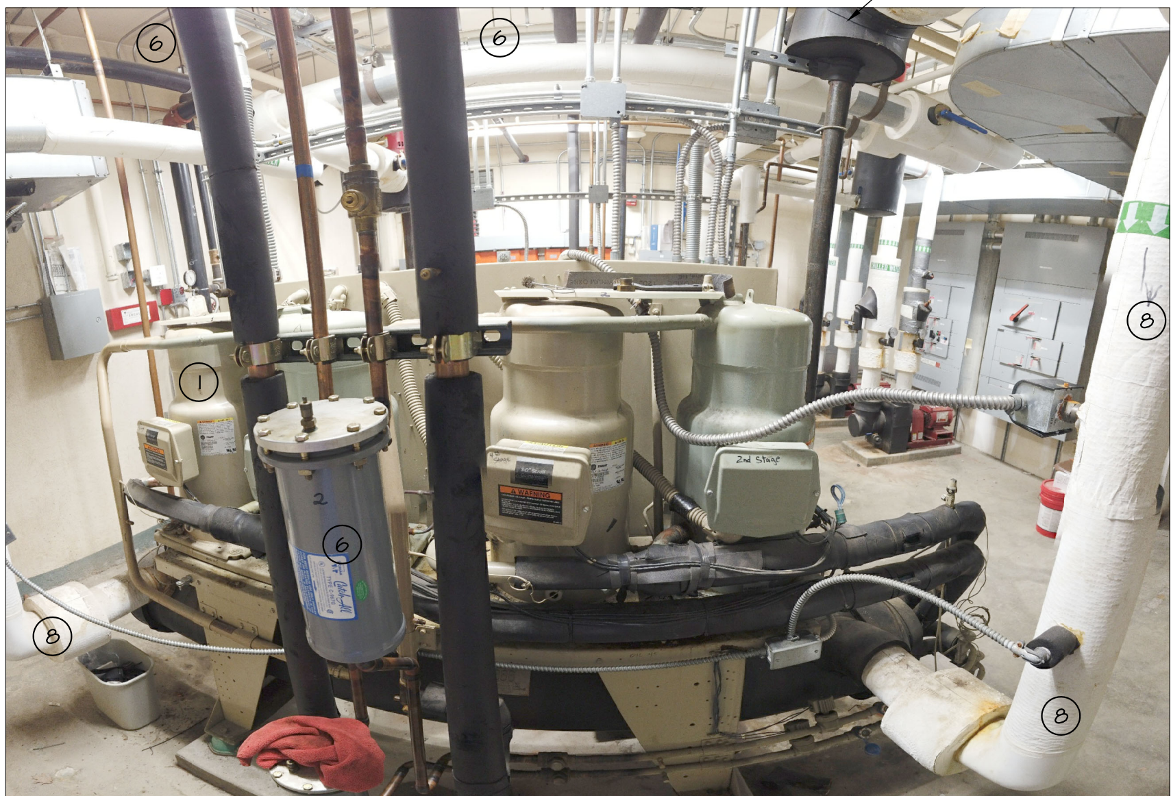
EXIST. CONDITION PHOTO #5
