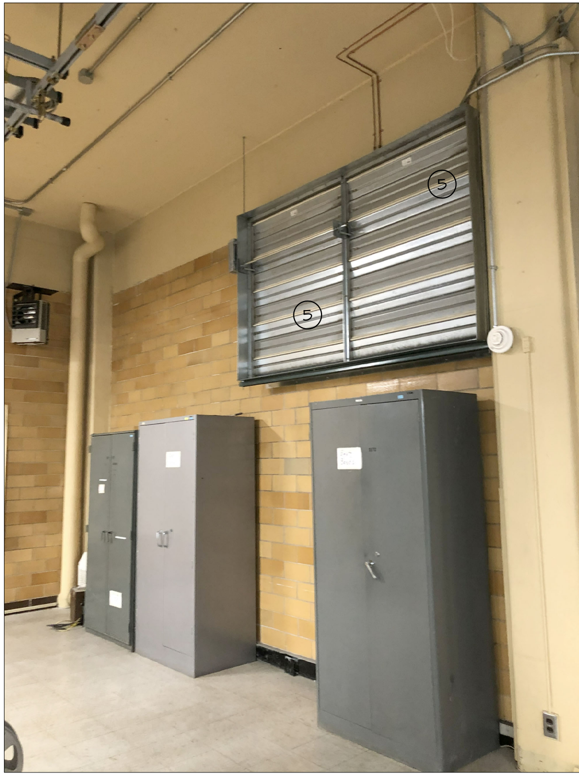
EXIST. CONDITION PHOTO #15
