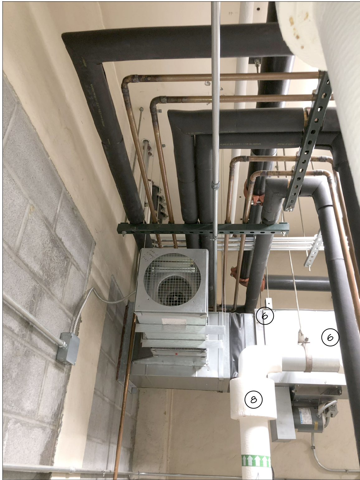
EXIST. CONDITION PHOTO #8
