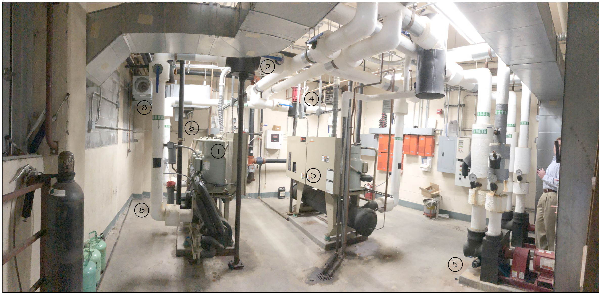
EXIST. CONDITION PHOTO #2
