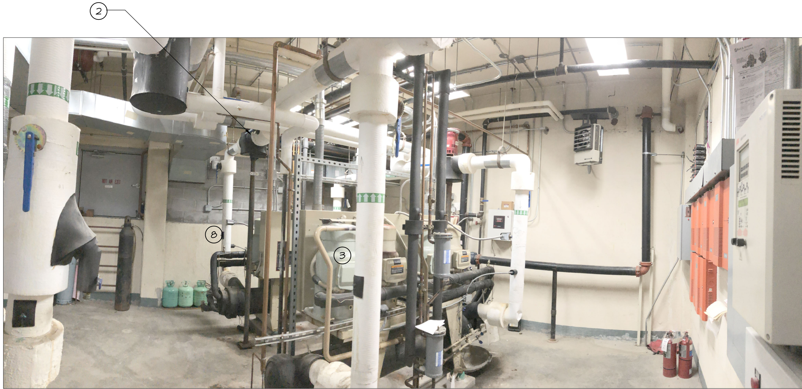
EXIST. CONDITION PHOTO #7
