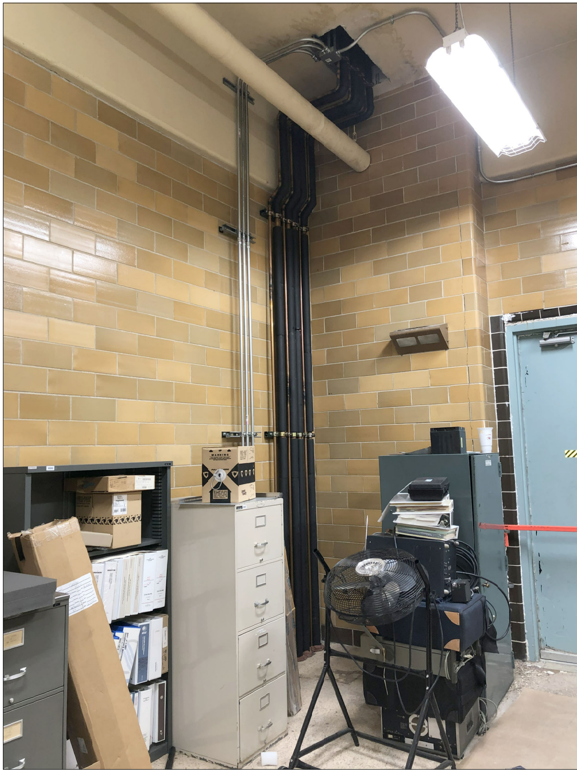
EXIST. CONDITION PHOTO #11
