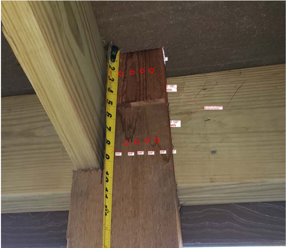
Fig. 1 – Middle Deck Post Connection with Lag Screws
