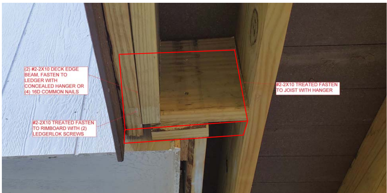
Fig. 3 – Deck Ledger Connection with LedgerLOK screws.
