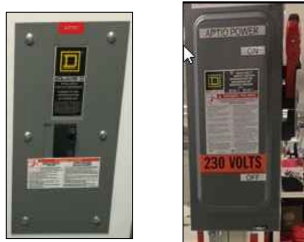
40 Amp breaker or 40 Amp Disconnect Switch
