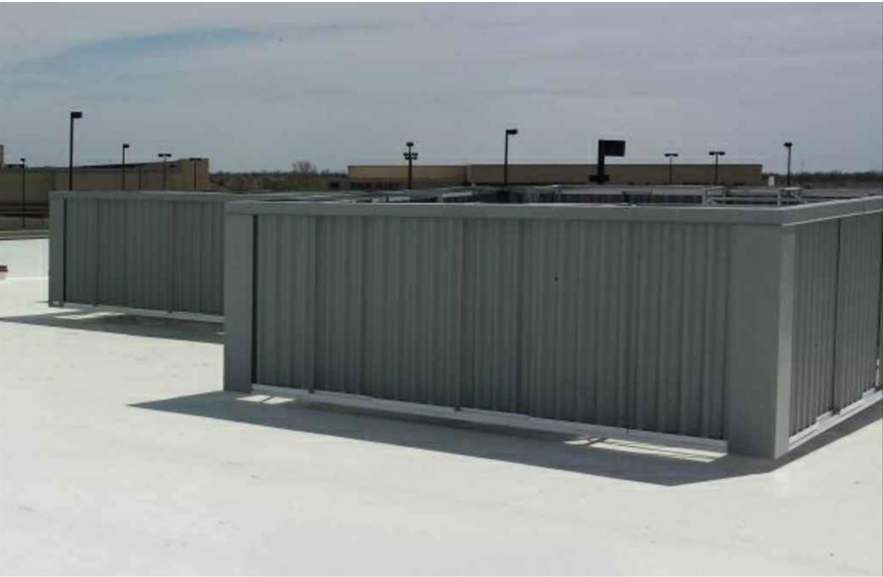
2 Screening of Rooftop Mechanical Units (Final determination of application will be made per ground level visual inspection.)
