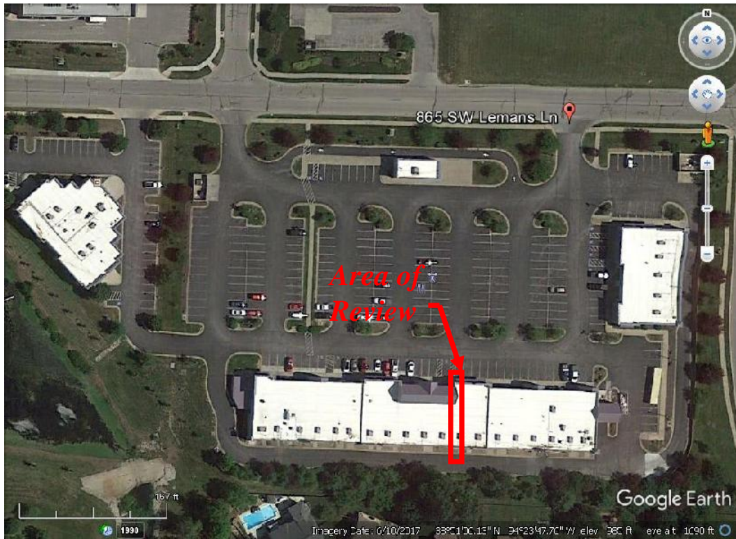
Site Aerial View – 06/10/2017
