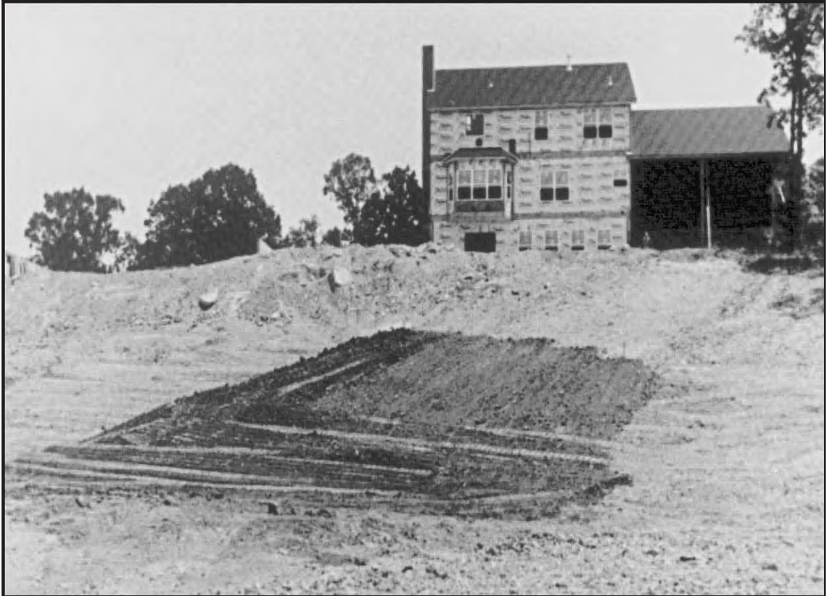
Figure 6.16 It's important to mix or incorporate topsoil with the underlying subsoil to prevent sloughing on sloping soils. Source: C. Rahm, NRCS. St. Louis Co.
