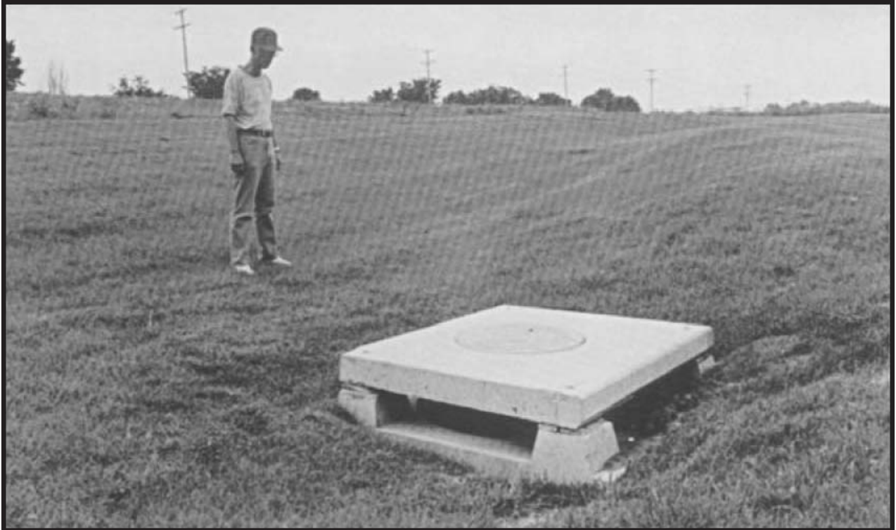
Figure 6.25 Permanent vegetation can be used to stabilize many structures, such as this grassed waterway, ensuring that runoff is relatively sediment-free.
