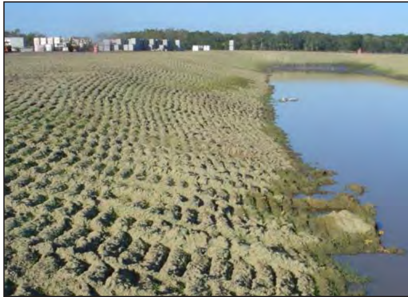
Figure 6.15 Track walking with a dozer up and down the slope provides horizontal grooves to reduce stormwater flow volumes and velocity therefore reduces potential for erosion of the slope. Source: ABC's of BMP's, LLC
