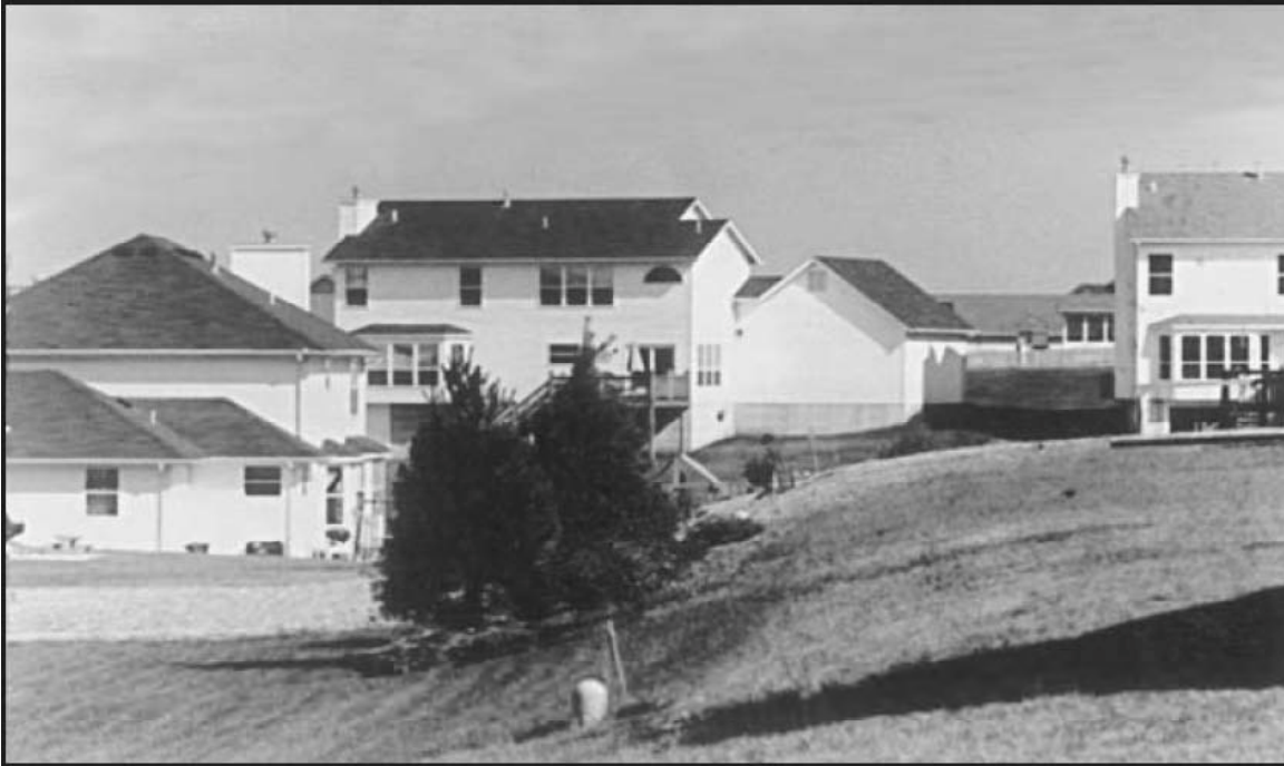
Figure 6.13 Lot benching can shorten slope length and prevent erosion while improving the homeowner's yard. Source: C. Rahm, NRCS, St. Charles County
