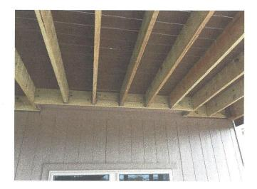
As shown in the photos above, a portion of the deck is attached to a 1' overhang. Generally, decks should not be attached to overhangs because there is no support directly under the rim board and this could cause the rim board to pull away since the only support is nails through the rim board into the overhang joists. In this case, the deck is attached to the rim board with
