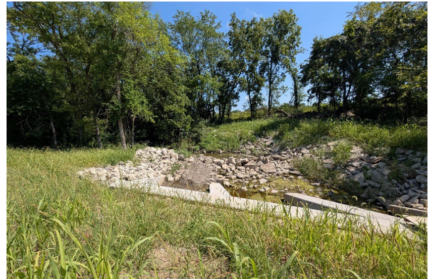
Photo 4 – Outfall 002 in Zone 3 – Clear discharge noted.
