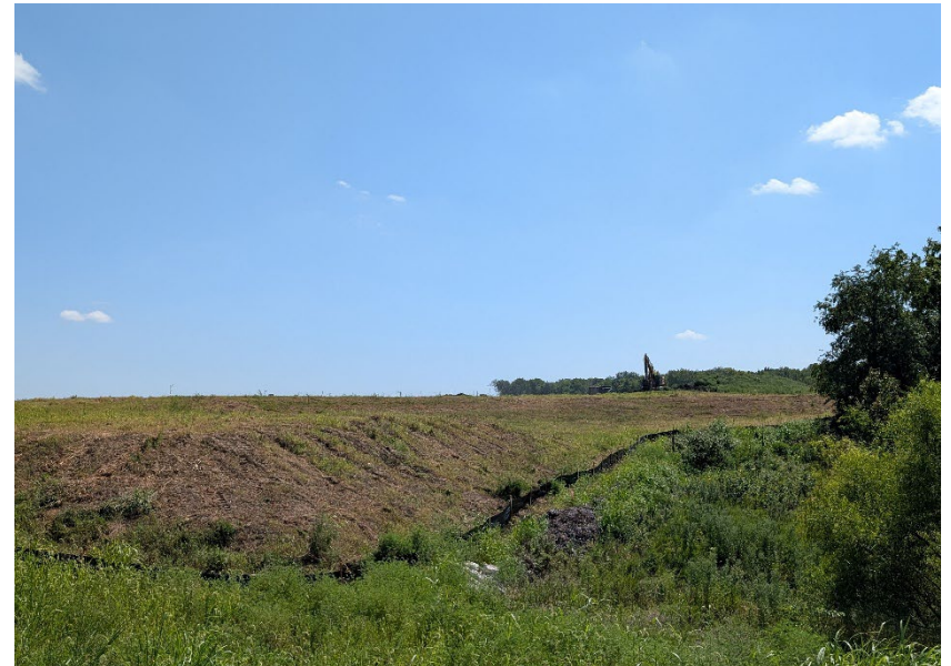
Photo 2 – Zone 1/Aria – Silt fence added, and grading activities started.
