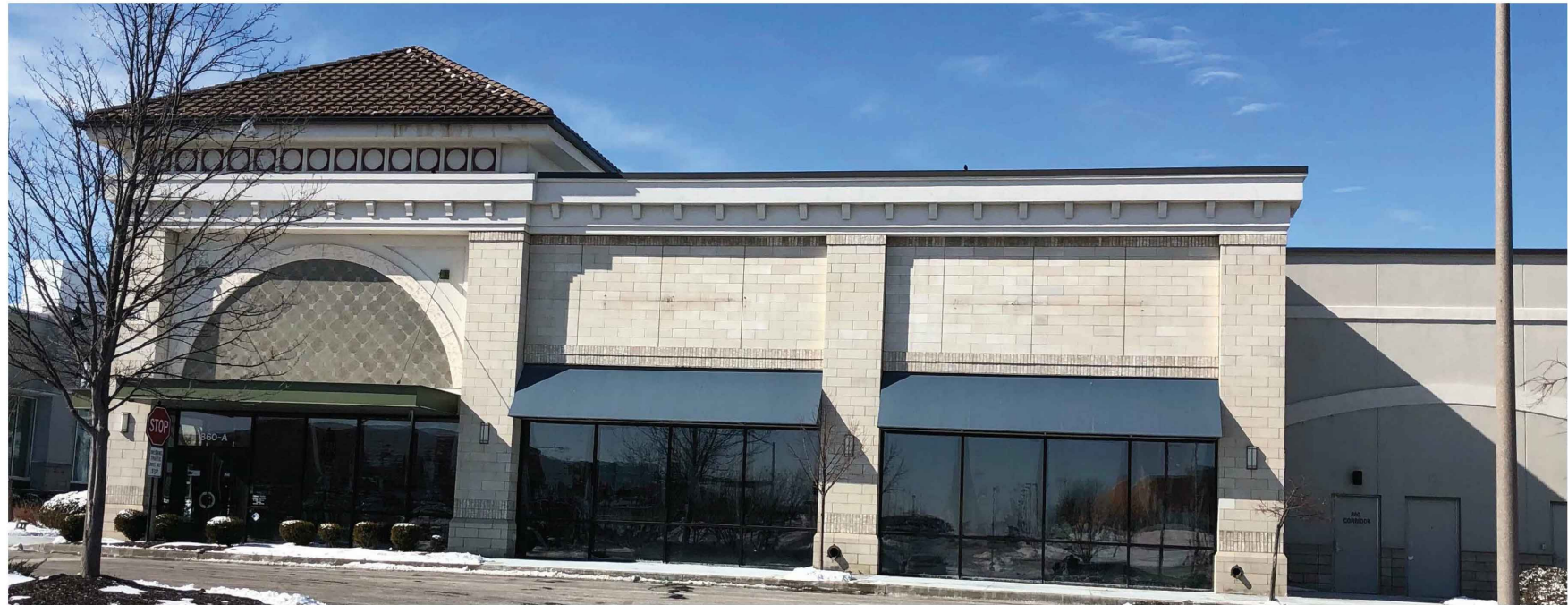
BEFORE - EAST ELEVATION
